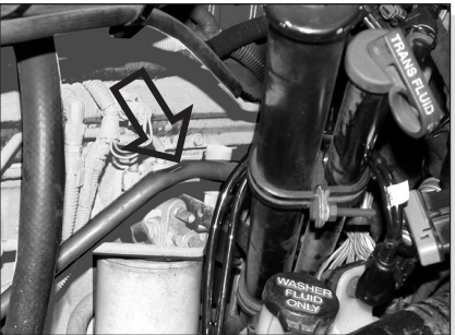
Damaged discharge line shown.
