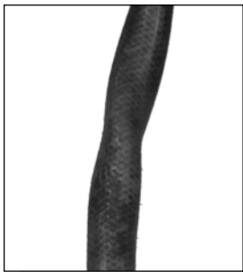
Partly collapsed inlet line shown.
